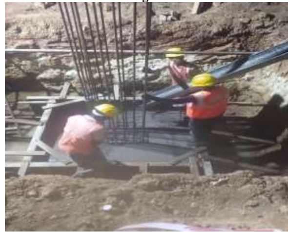
Footing Concrete Work, Pedestal Barbending & Shuttering
