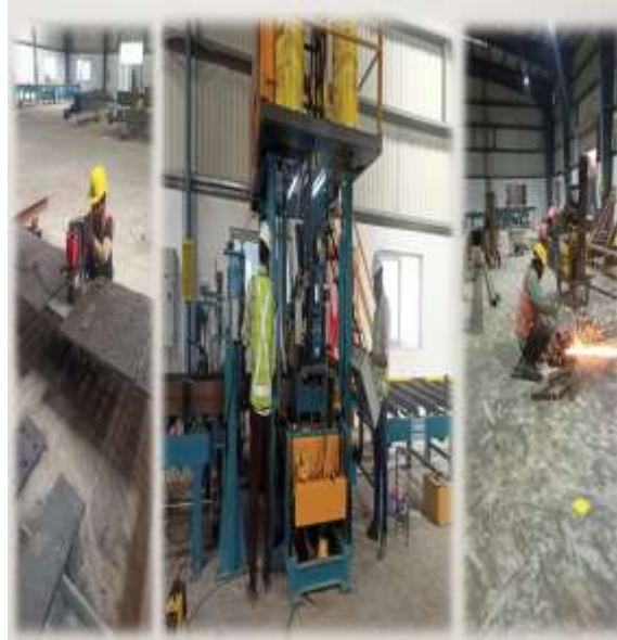
Civil Foundation Fabrication Work
