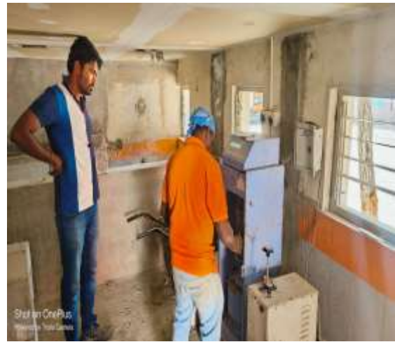
PCC Concrete Trial Mix Testing
