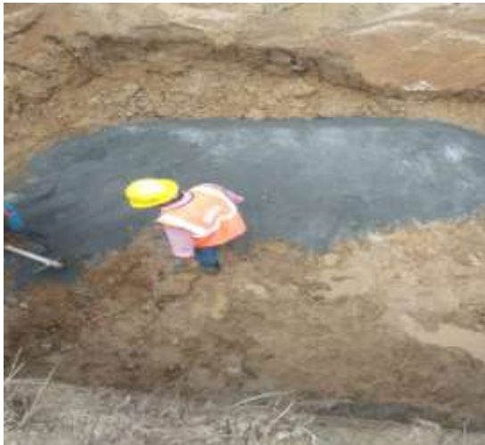
M- Sand Filling Work
