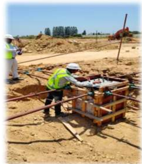
Anchor Bolt Fixing & Checking
