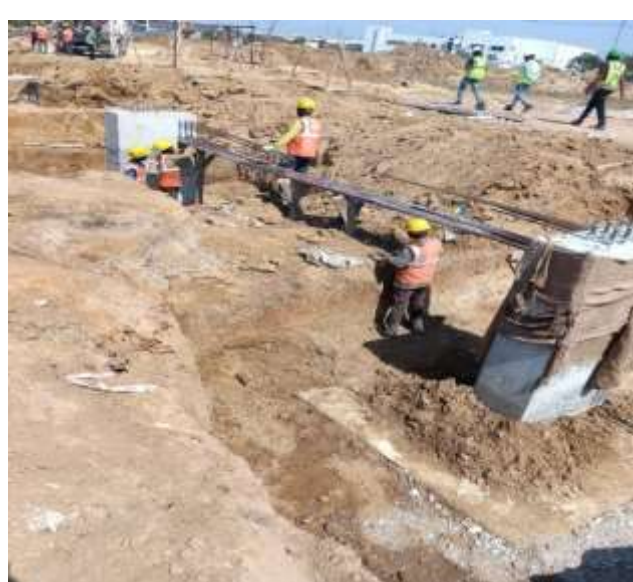
Plinth Beam Shuttering and Concrete Casting
