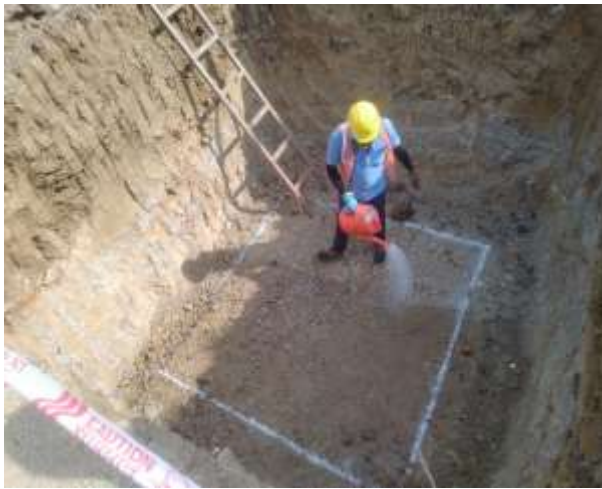
Anti Termite Work
