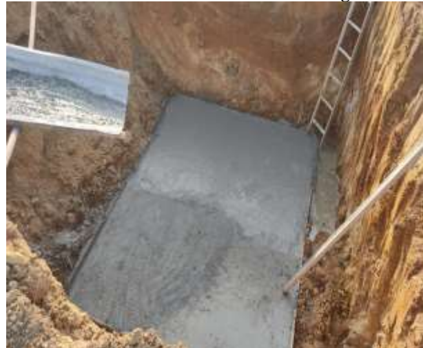
PCC Concrete Work
